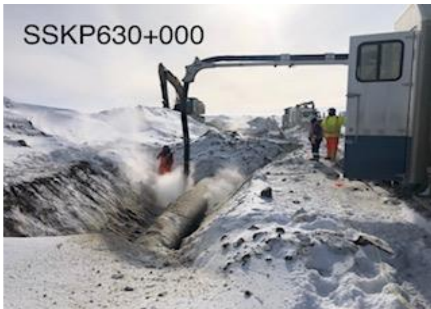
Hydro Vac clearing snow from pipeline
