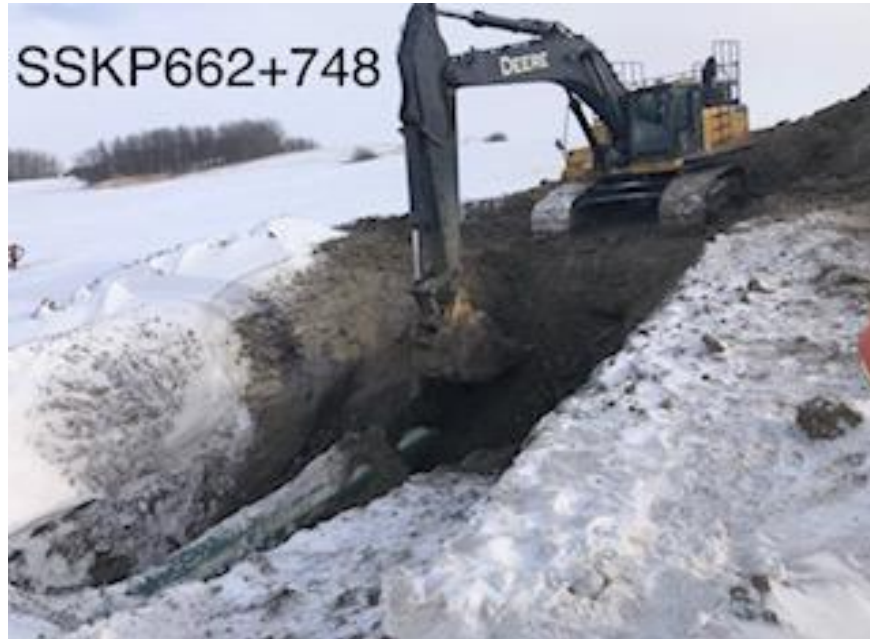
Ovality excavation S111 SSKP662.748
