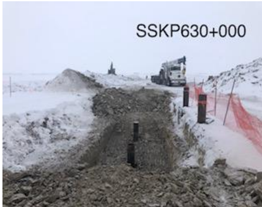
MLBV16 Cleared around the piles background backfilling mainline downstream of valve site
