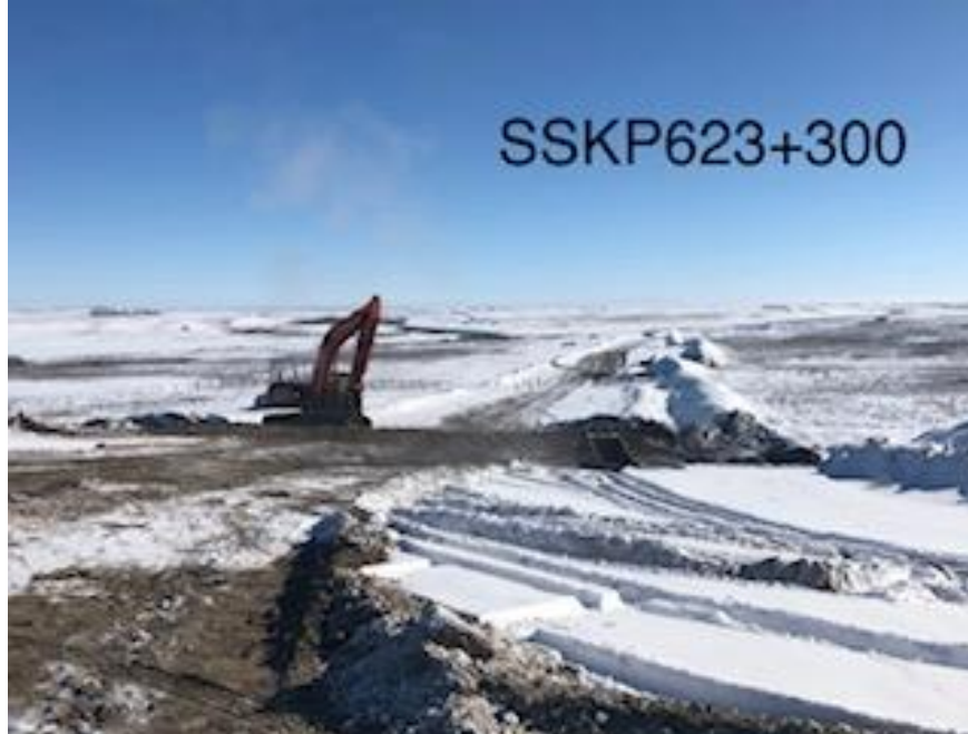
Diversion berms being installed at Chapleau Lake HER132
