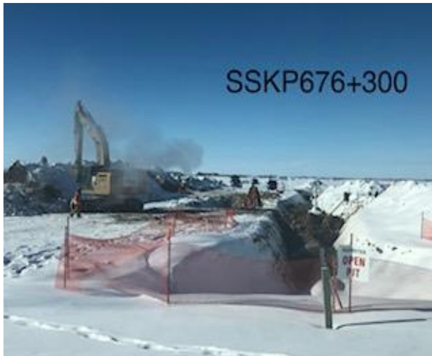
MLBV17 shade and backfill of upstream and downstream of valve site
