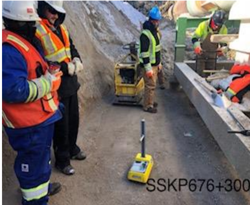
MLBV 17 compaction testing inside open pit area
