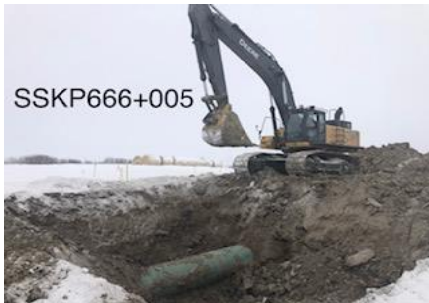
Ovality S152 excavation in wet land crossing SK598
