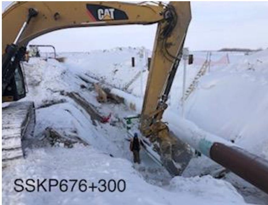
MLBV17 Cleared snow from trench line – SF80 west
