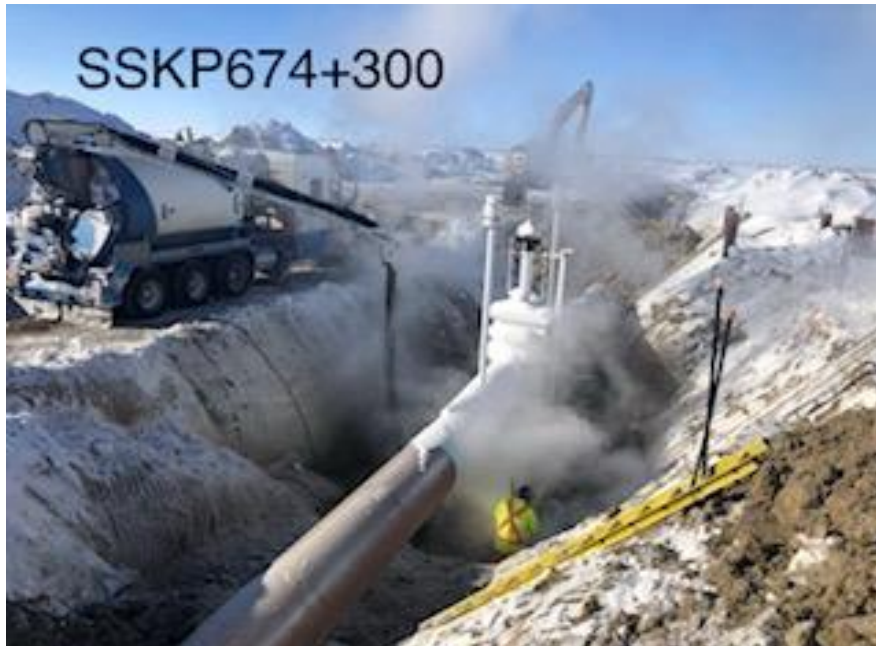
MLBV17 Hydro vac operator removing water from underneath pipeline before compaction
